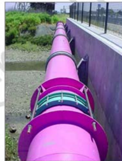
Figure PW-4a: Recycled water distribution line from Clovis, CA. Image Credit: Sherwood Design Engineers
